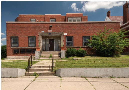
Pre-renovation of The Manse exterior
