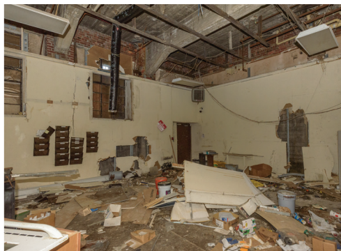
Pre-renovation of the Ballroom
